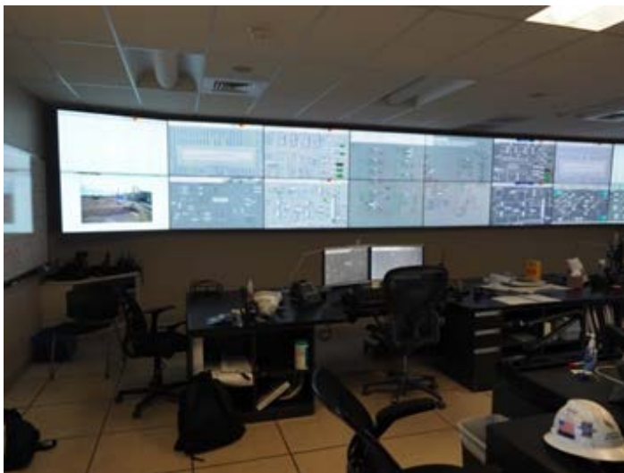
Lancaster Facility control room
