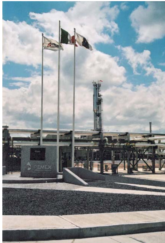
Figure 1 – Pemex CPG Burgos Plant 1
