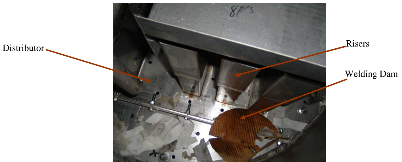
Figure 7 – Top Deethanizer Distributor
