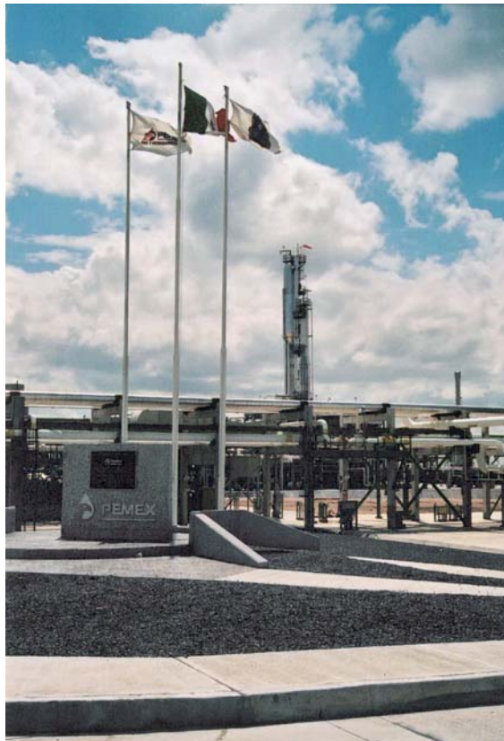
Figure 1 – Pemex CPG Burgos Plant 1
