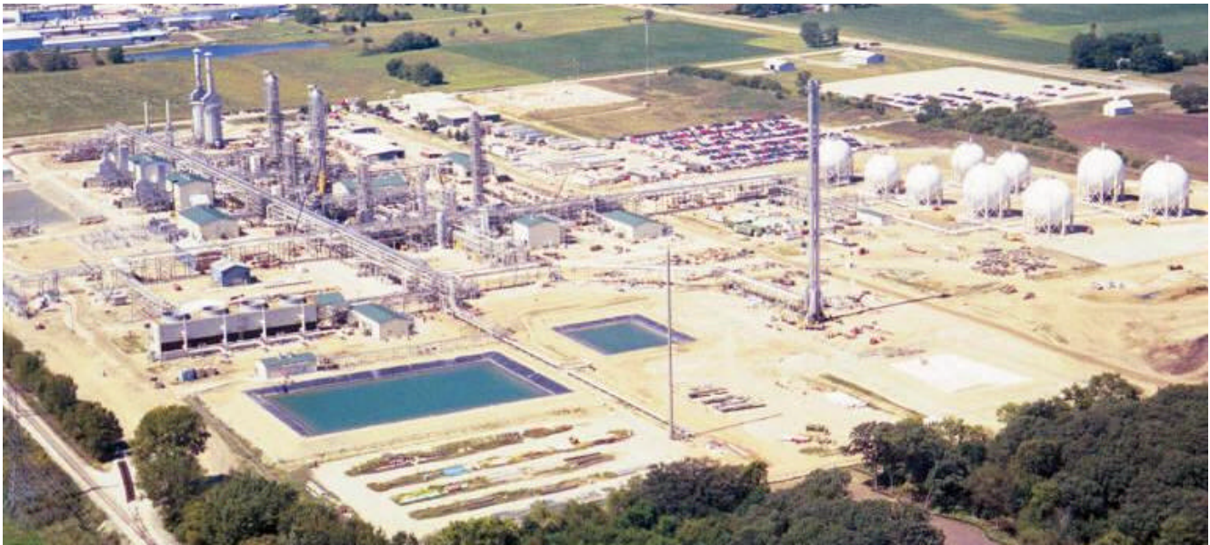
Figure 2 – Aux Sable NGL Recovery Plant
