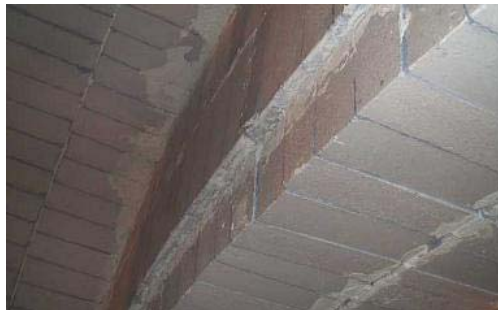
Figure 7. Non-Anchored Flatwall Brick
