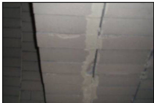
Figure 9. Displaced Bullnose Brick
